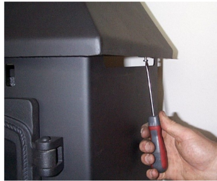
Figure 10: Tightening The Canopy
